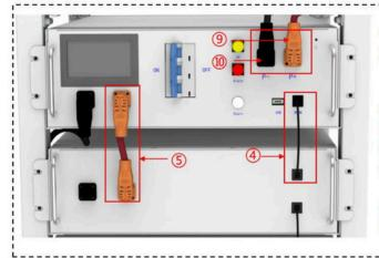
control box Connect B+ to battery pack B+ using cable ⑤.
